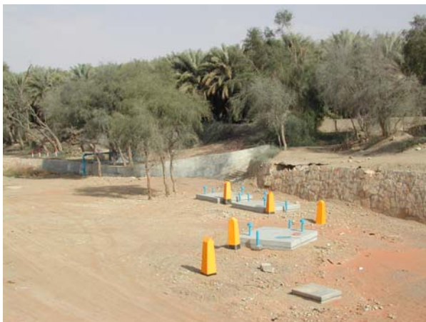
Desalination support pipeline for Al Aini and Al Daoudi Falaj
