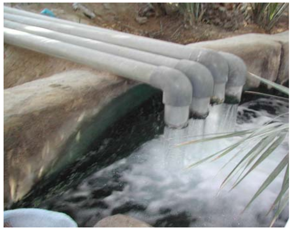
Al Mutared source wells discharge
