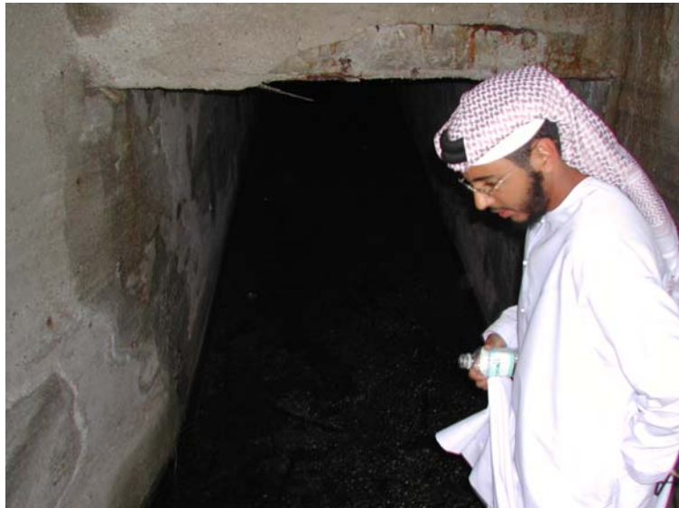
Figure 11. Sub-surface Falaj type channel at Ayn Al Fayda
